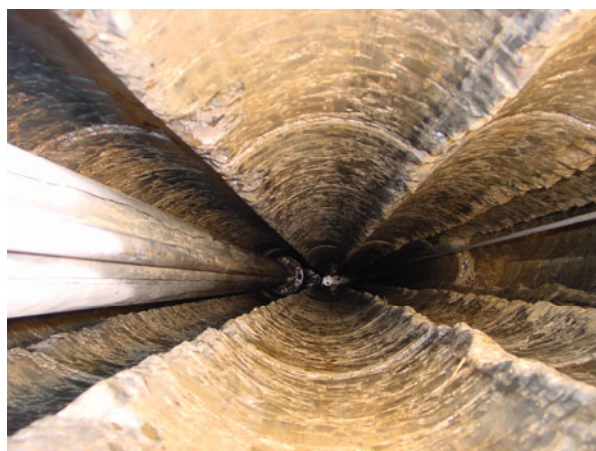
Figure 10. Downhole photograph of overlapping drill holes
